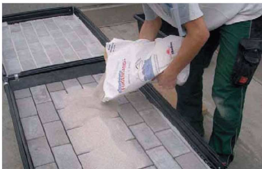
Figure 1: Applying the grout (Photo taken on 21.01.2010)
