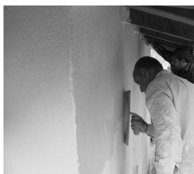
**Warnings:** during the choice of the paint it's important to remember that finishing plasters and wall paints with a value of widespread reflexion inferior to 20 are not suitable for external thermal insulation systems. Execute the application following the technical data sheet instructions and the producer' indications for the chosen finishing.
